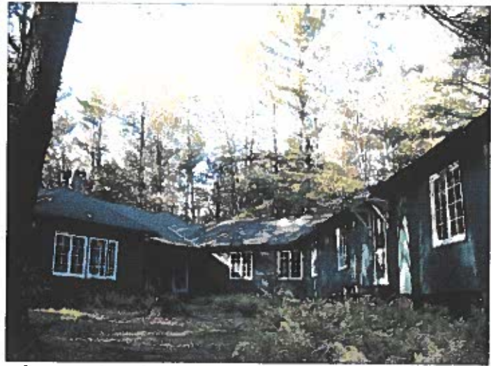
Camp –view from rear –large pines surrounding
